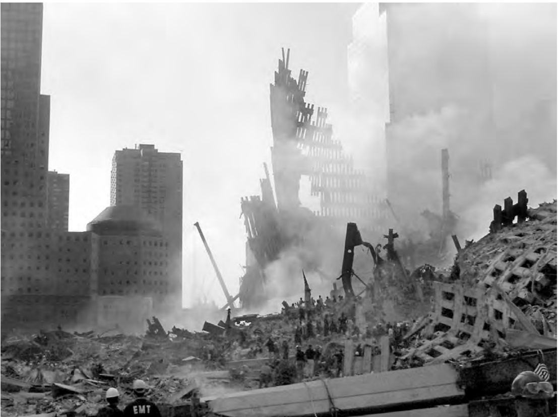
Smoke clouds the remaining structure at ground zero, the site of the World Trade Towers destroyed in an attack on September 11, 2001. (U.S. Air Force)
